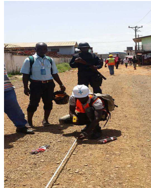
Establishing centerline
