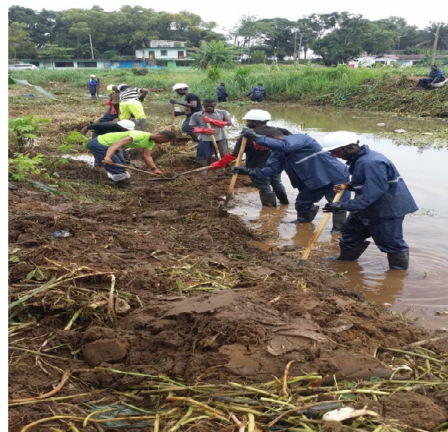
Quick impact project to avoid continual flood of water in the communities
