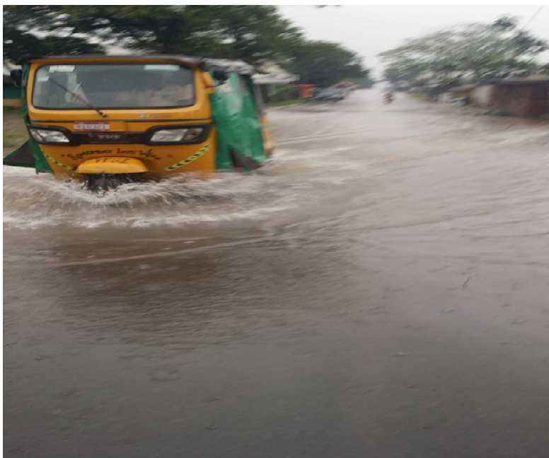
Flooded Carriageway due to clogged drainages
