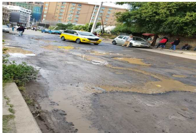
Poor design of drainage
