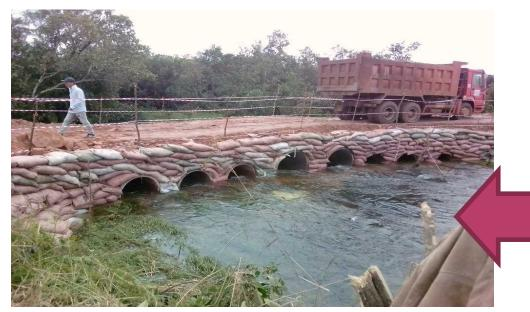
THE CONSTRUCTION OF A DIVERSION IMMEDIATELY COMMENCED SO AS TO ALLOW THE FLOW OF TRAFFIC AS A SHORT TERM INTERVENTION.
