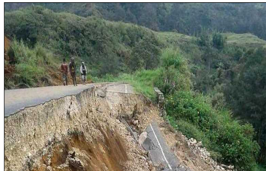
Slippage of embankment by seismic action/internal failure
