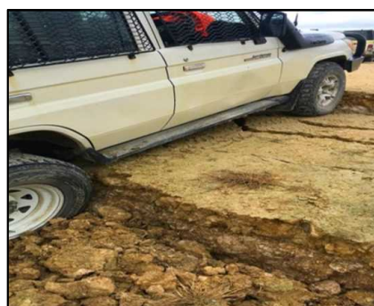
Slippage of embankment by seismic action/internal failure
