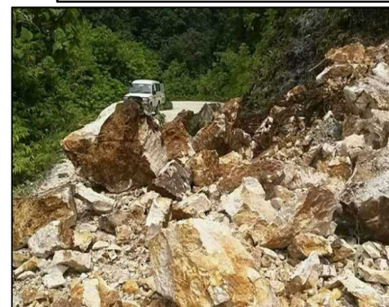
Slippage of embankment by seismic action/internal failure
