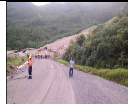
Slippage of embankment by seismic action/internal failure
