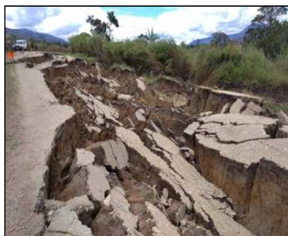
Slippage of embankment by seismic action/internal failure
