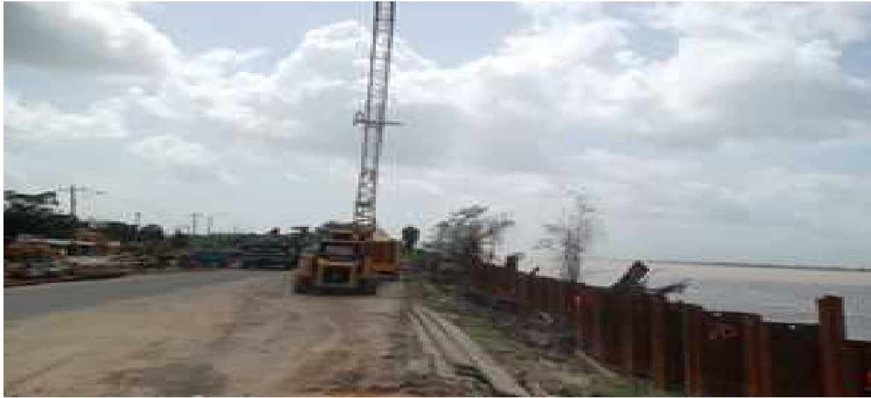
STEEL SHEET PILE REVETMENT 鋼板杭の設置
