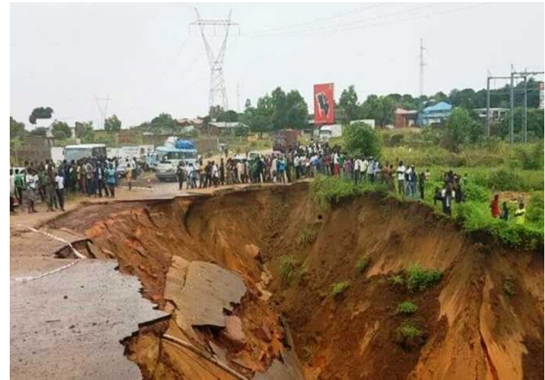
Slope failure in RN 1 after heavy rain 豪雨後のRN 1の斜面崩壊
