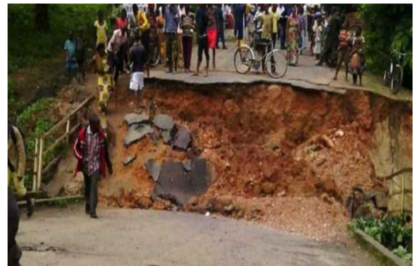
Slope failure in RN 1 after heavy rain 豪雨後のRN 1の斜面崩壊
