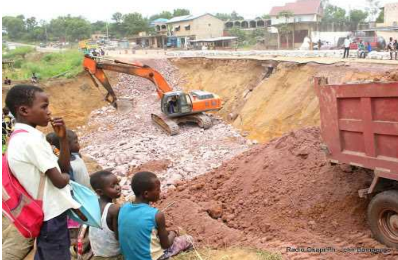
Better geotechnical knowledge and good choice of materials より良い地盤工学的知識と材料の良い選択
